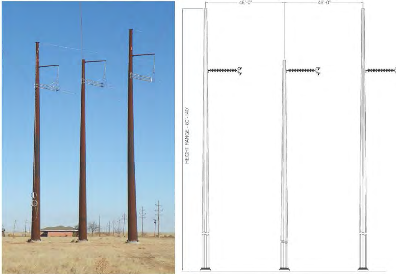
Figure 2-4 Typical Steel Three-Pole Angle Transmission Structure
