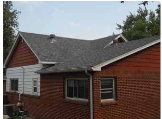
Roof looking east
