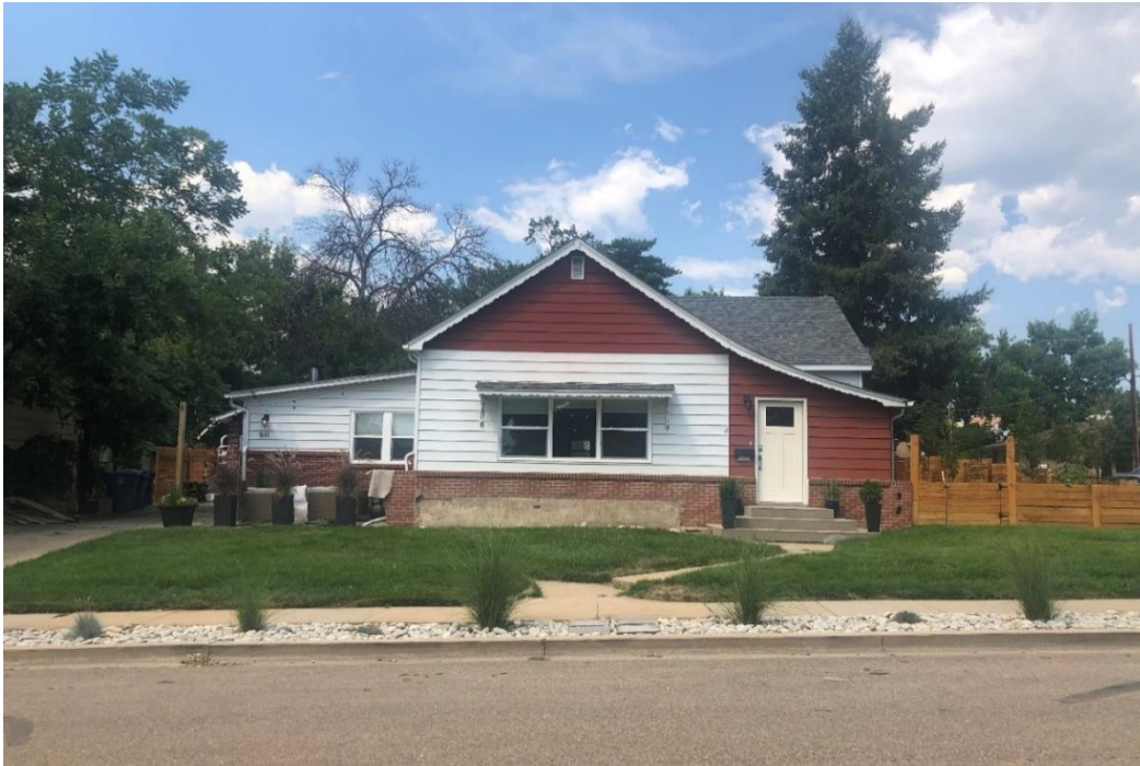
841 Jefferson Avenue, East view. 2020.
