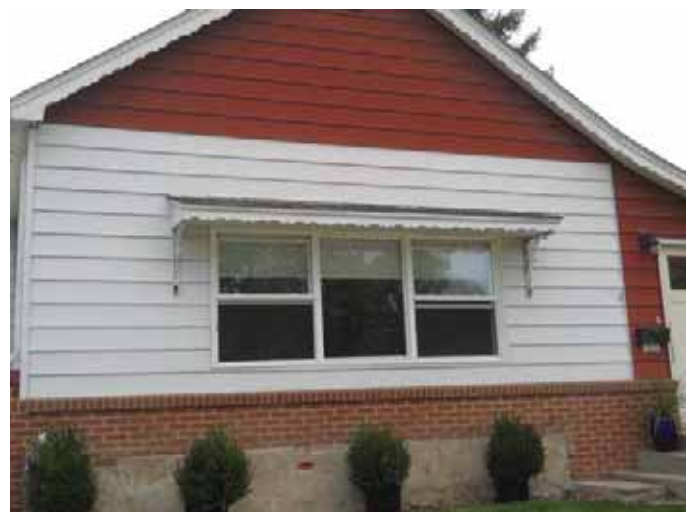
Exterior wood trim and shed roof
