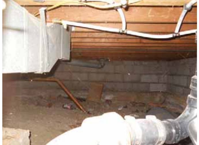
Foundation and crawlspace
