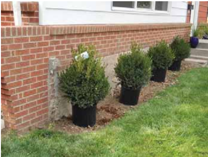
Removed attached garden boxes
