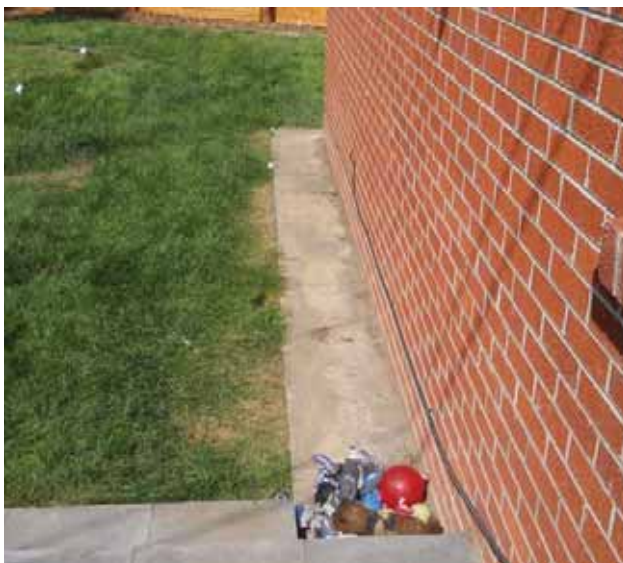
Concrete at building perimeter
