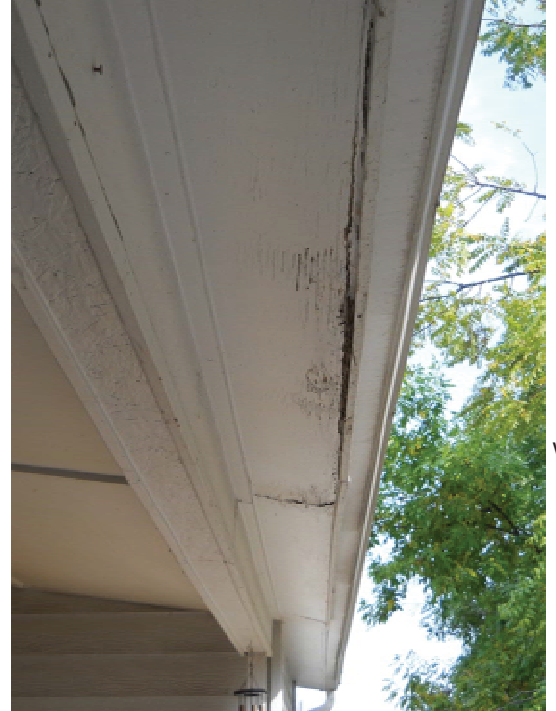
Deteriorating soffit at gutter joint
