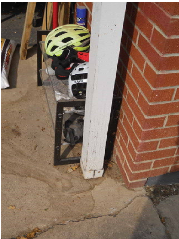
Covered porch supports
