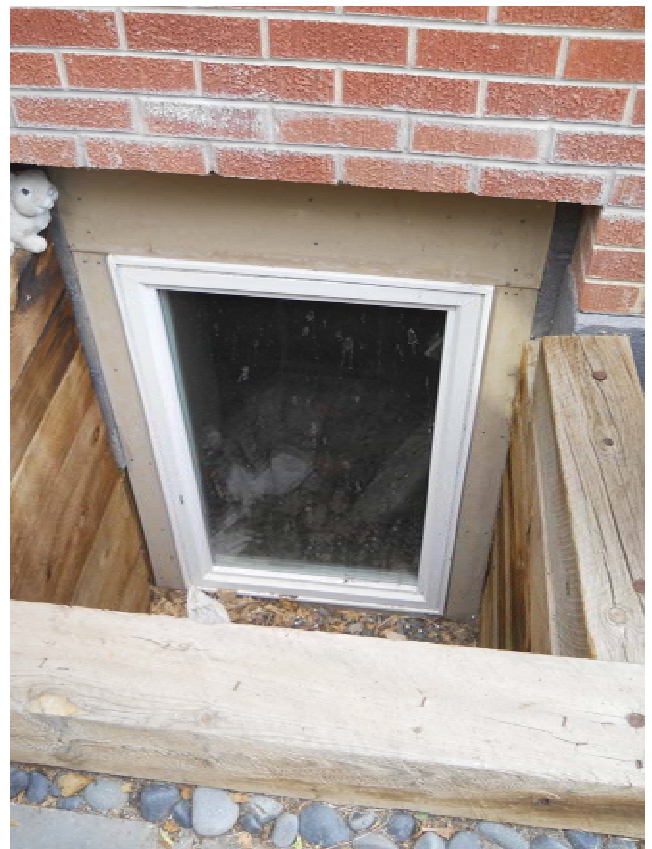
Egress Basement Window
