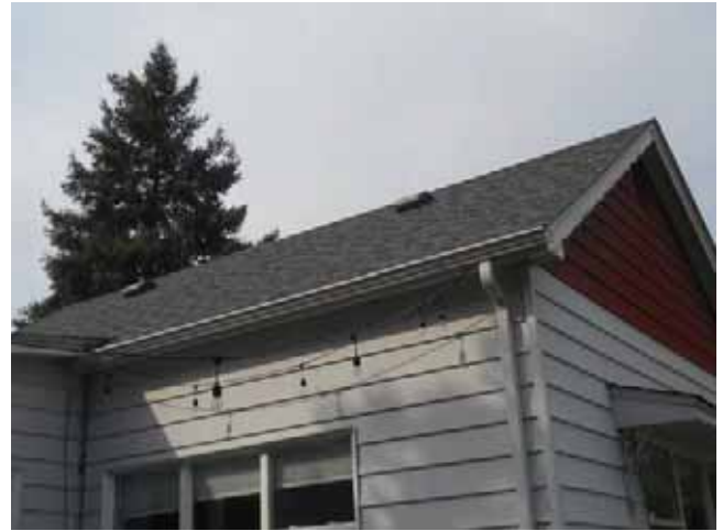
Roof, looking north
