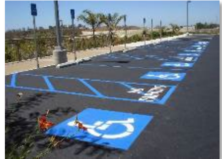
Example: ADA compliant striping (surface lot)
