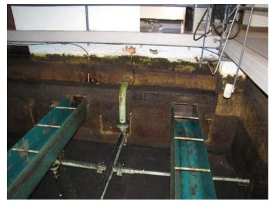
Figure 8. Spalling and exposed reinforcing in Filter 2.
