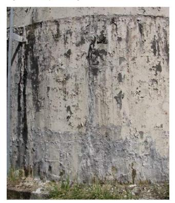
Figure 10. Map cracking at tank exterior.
