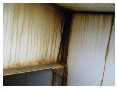
FIGURE 14 Columbia View Reservoir Roof Beam and Roof Plate (looking through roof hatch)
