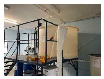
Figure 16. Filter aid polymer day tank.
