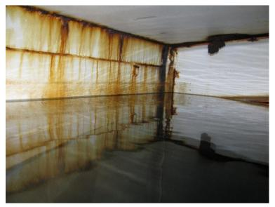
FIGURE 9 Sorosis Reservoir Roof Beam and Roof Plate (looking through roof hatch)
