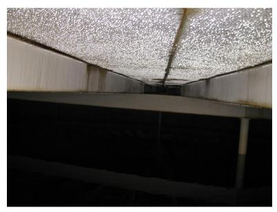
FIGURE 15 Columbia View Reservoir Roof Beam and Roof Plate (looking through roof hatch)
