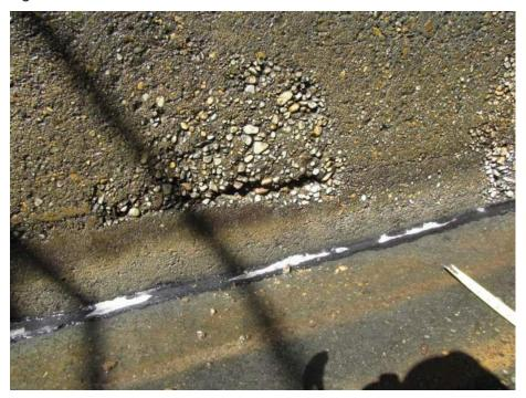
Figure 3. Interior of Sedimentation Basin 2 at base of wall.
