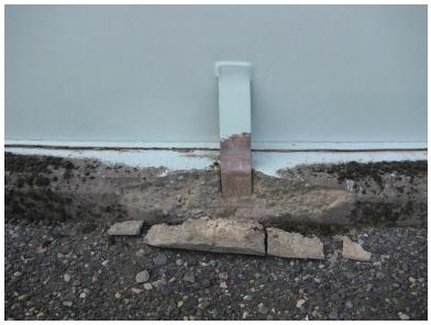
FIGURE 13 Columbia View Reservoir Base of Tank Anchors
