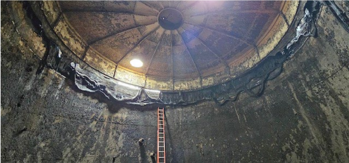
Interior of Digester 1: Before and after removing the cover.
