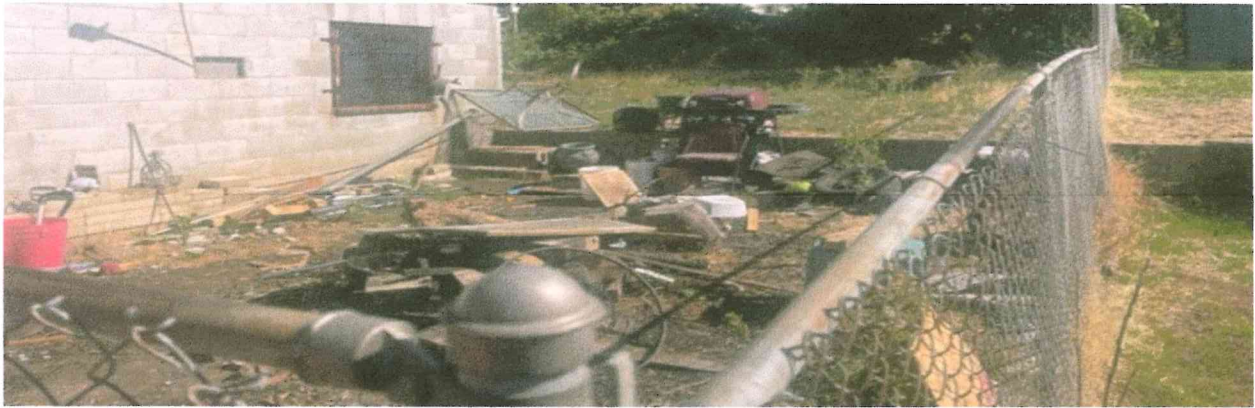
08/10/2023 ABATEMENT pics for 1212 East 10 th Street
