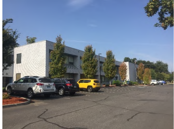
A view of the subject from the northeast corner
