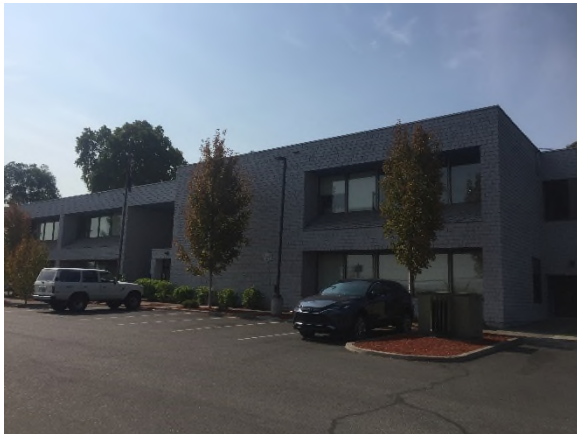
A view of the subject from the northwest corner
