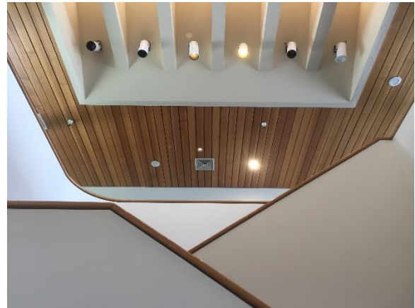
Lobby ceiling & stairs
