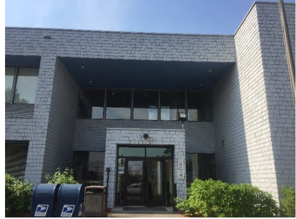
Main entrance exterior
