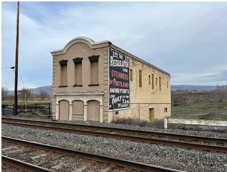
Photo 6: Exterior from SE corner
