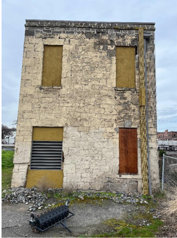
Photo 3: North exterior elevation
