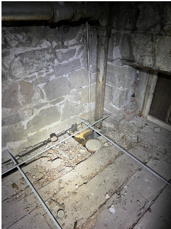
Photo 16: NW corner – viewed from interior
