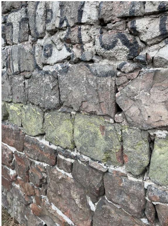
Photo 8: Exterior stone and mortar joints
