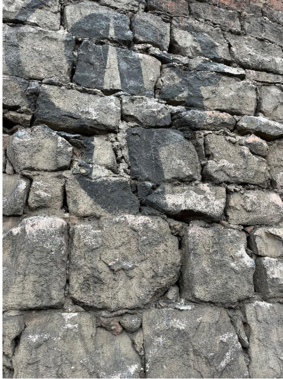
Photo 7: Exterior stone and mortar joints
