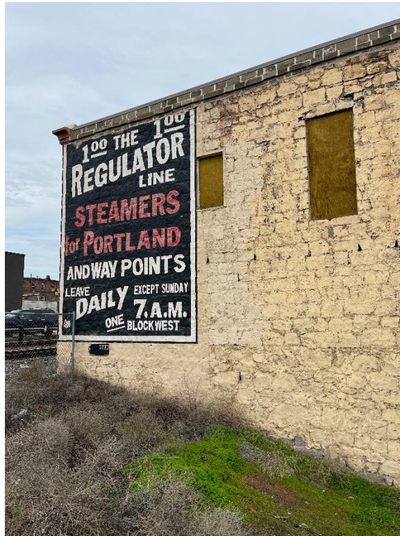
Photo 5: South end of east exterior elevation
