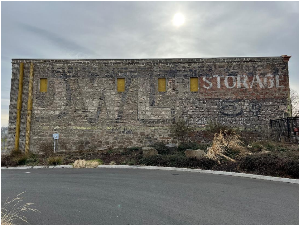
Photo 2: West exterior elevation
