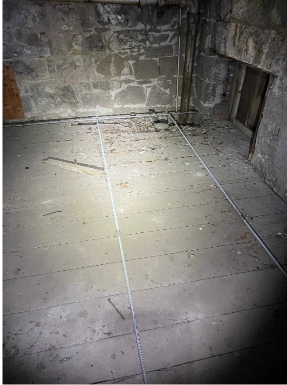
Photo 15: NW corner – viewed from interior
