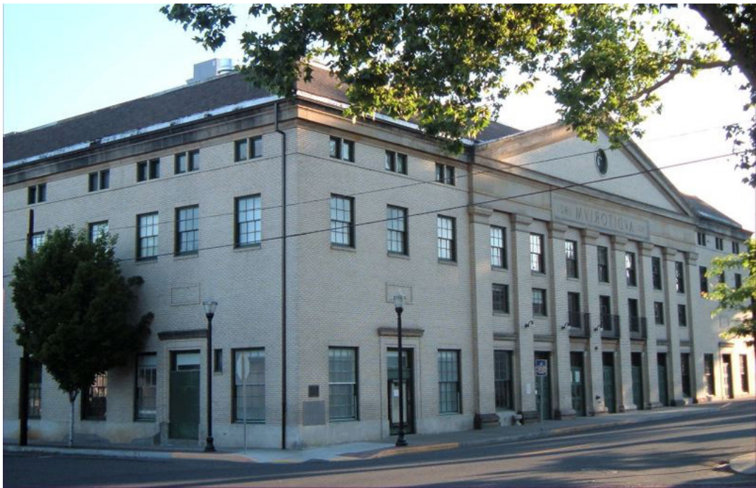
Proposed new windows along second floor of building to be single-sung steel sash featuring divided lights with spacer bars. consistent with historical style as seen at the Dalles Civic Auditorium Building above (Constructed 1922)
