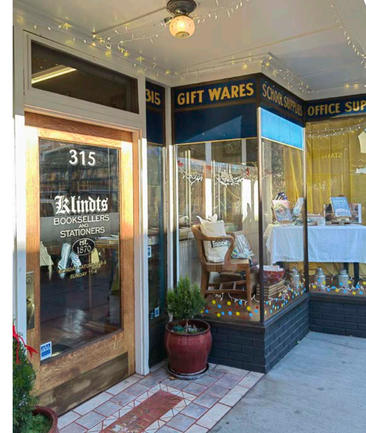
painted brick storefront, tiled entry, gold-leaf signage, boxed eave, Klindts on 2nd street, est. 1870
