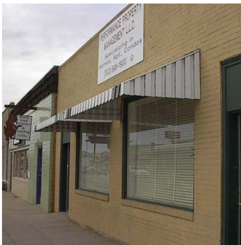
Example of an undesirable typical residential metal awning Illustration 5.5.7.g7
