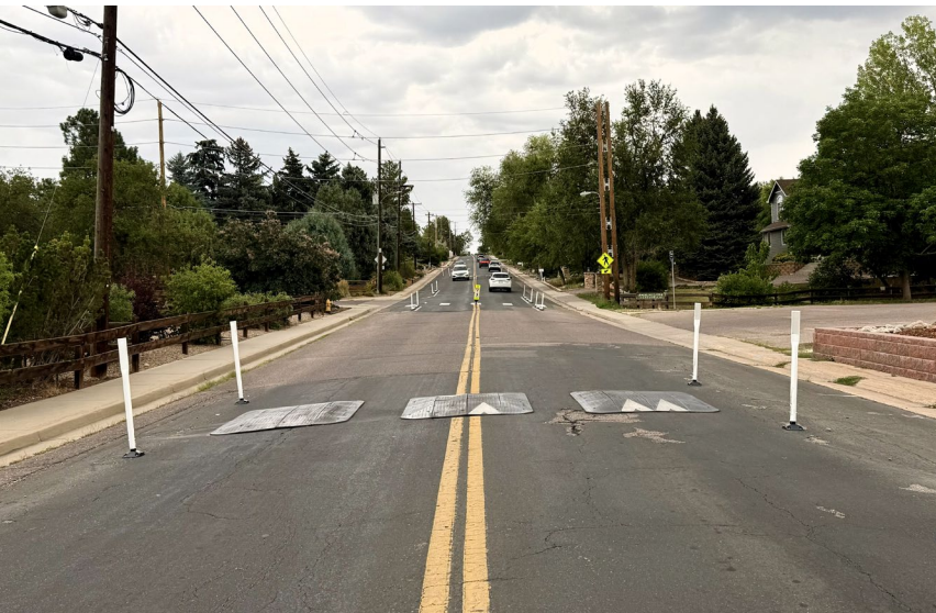
Caley Ave. & Datura St. speed cushions
