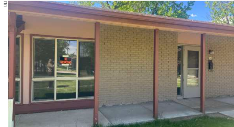
Now vacant, Geneva Village is a 28-unit complex of apartments designed by noted architect Eugene Sternberg.
