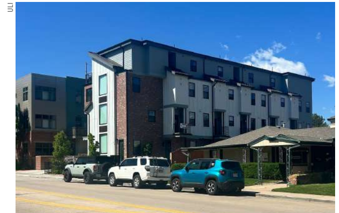
Nearby residential on Prince
