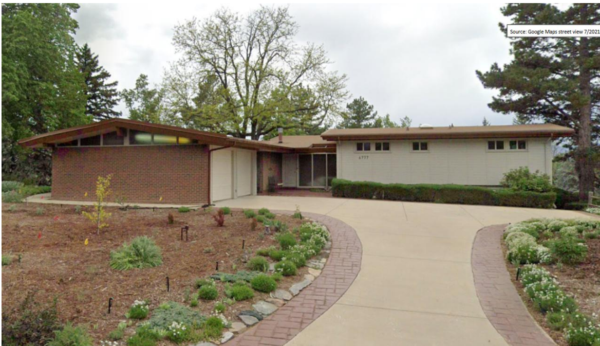
Figure 3: View of the front façade of the home from Southridge Lane looking to the southwest
