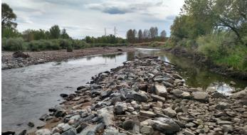
Photo example on the left shows the narrowed channel and desired bank materials prior to the flood, and some of the scour and loss of sediment this project request will repair.
