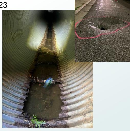
Replace 1200LF new storm sewer, repair street, new outfall alignment
