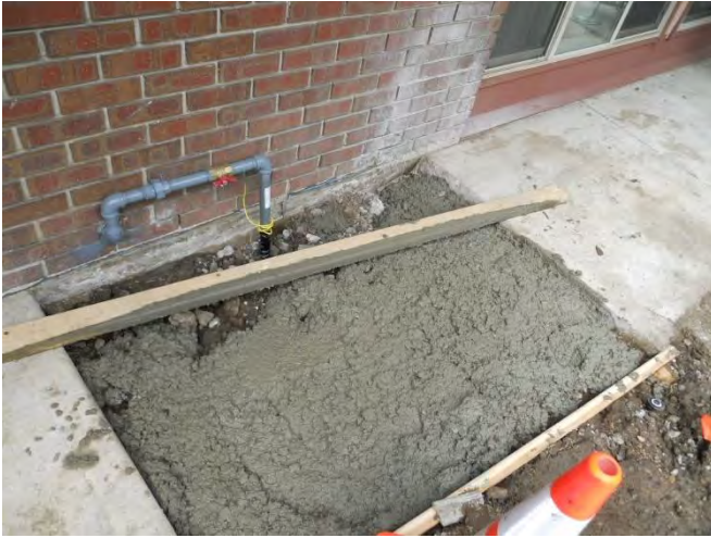
109. Natural gas line service replacement
