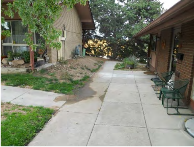
61. Area of settling concrete located between Building #3 and Building #2
