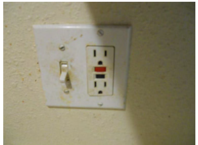
92. Typical apartment unit GFCI outlet
