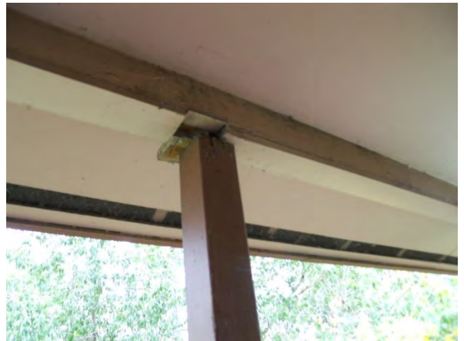
72. Building #3 rear roof overhang supports where detached
