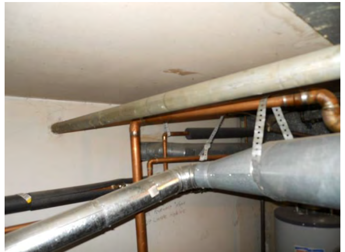
96. Exposed copper supply plumbing
