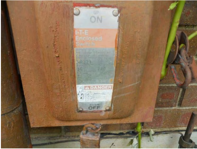
85. Zinsco main service electrical connection box labeling
