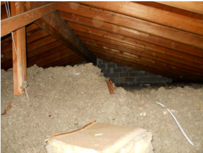
67. Typical attic roof framing, sheathing and insulation detail
