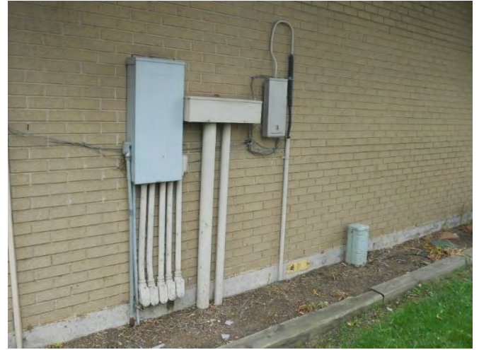
86. Typical upgraded apartment building General Electric electrical main service panel
