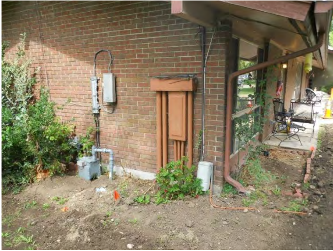
93. Typical apartment building Zinsco Electrical main service
