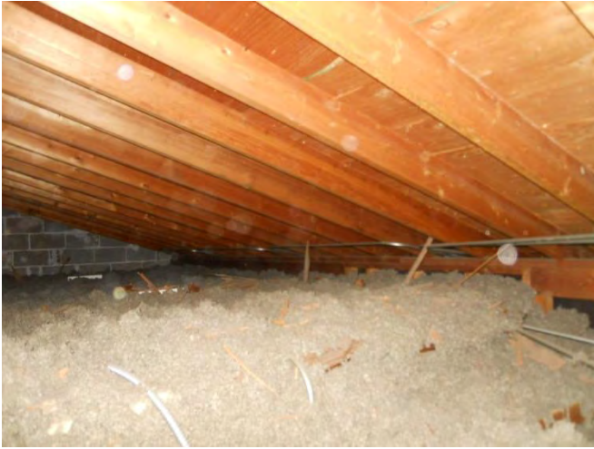
69. Typical attic roof framing, sheathing and insulation detail
