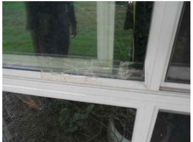
76. Damaged unit window on the upper window in the Function Room
