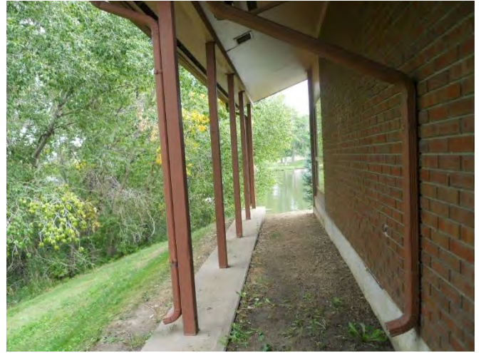
70. Building #3 rear roof overhang supports where detached from slumping concrete pad
