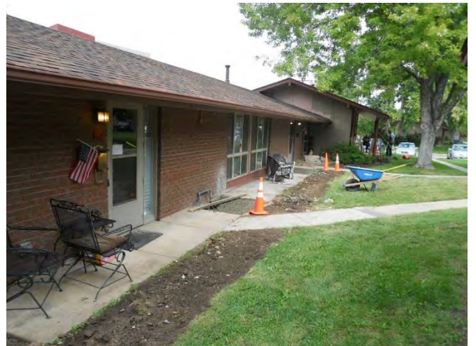
108. Natural gas line service replacement
