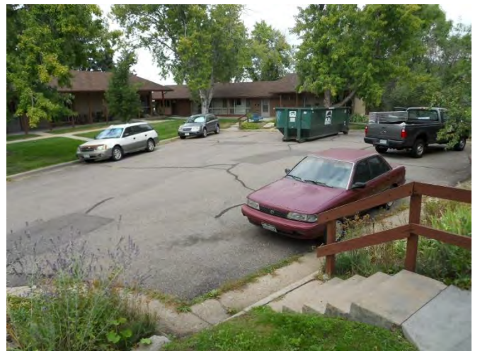
48. Onsite asphalt condition
