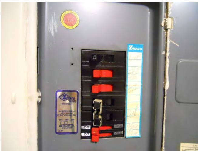
91. Typical apartment unit breaker
