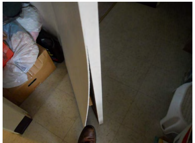
80. Delaminating apartment interior closet door
