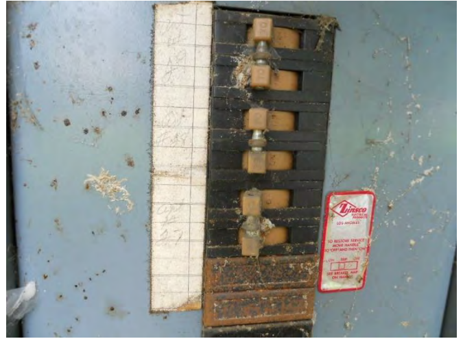
94. Typical apartment building Zinsco Electrical main service, 70 amps to each unit
