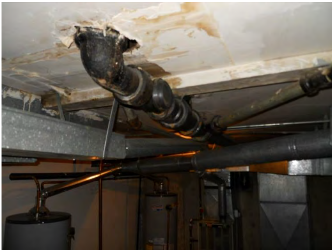
95. Exposed cast iron waste plumbing
