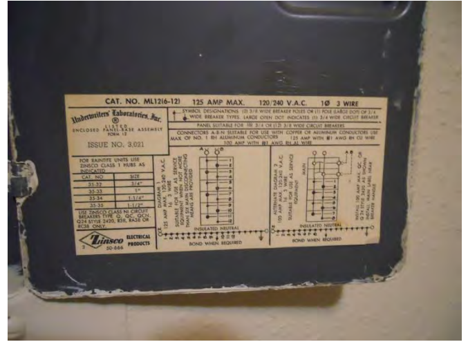
90. Typical apartment unit breaker panel manufacturer information
