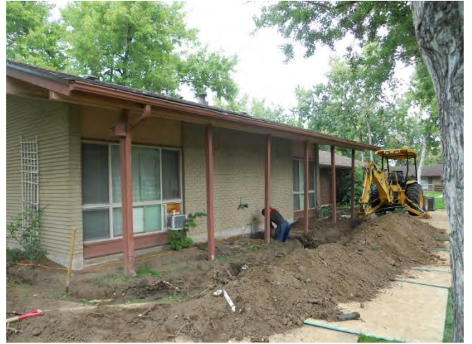
106. Natural gas line service replacement
