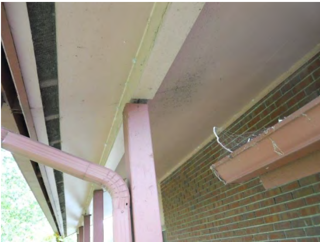
71. Building #3 rear roof overhang supports where detached
