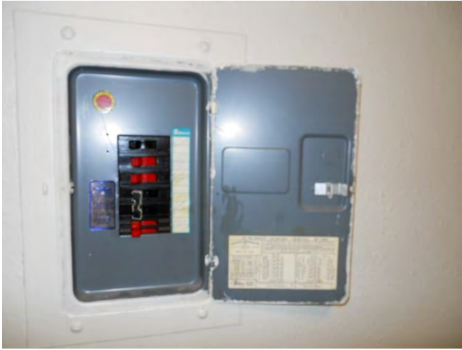
89. Typical apartment unit breaker panel
