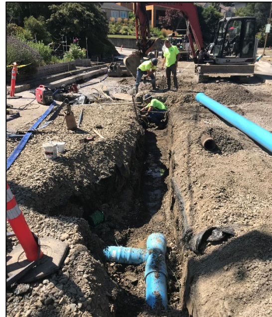
Wastewater service lateral installation
