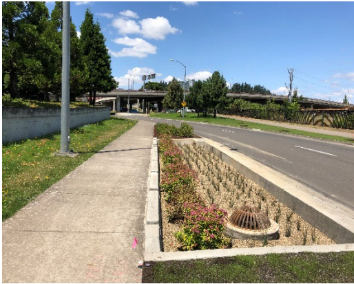
Stormwater planter on Hilyard Street
