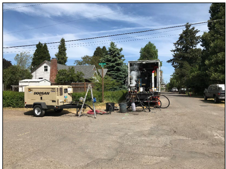
Lining a wastewater pipe
