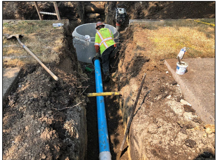
Wastewater manhole and pipe installation
