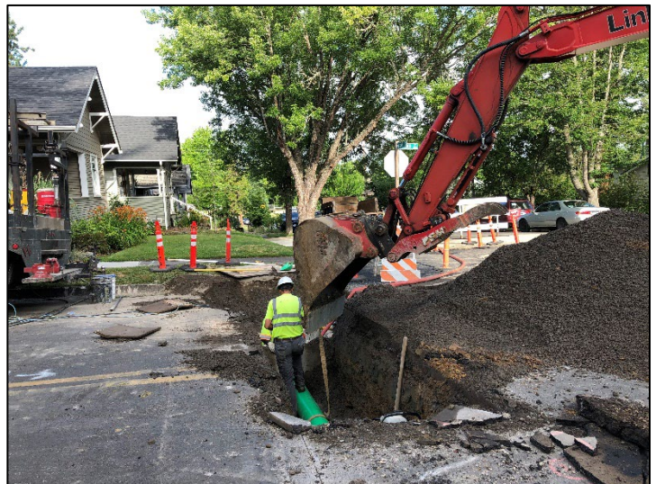
Installing stormwater pipe
