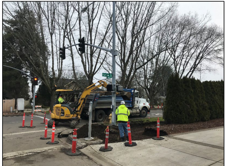
Sidewalk Access Ramp Construction on Harlow Road
