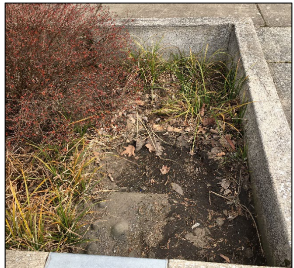
Sediment in a stormwater planter
