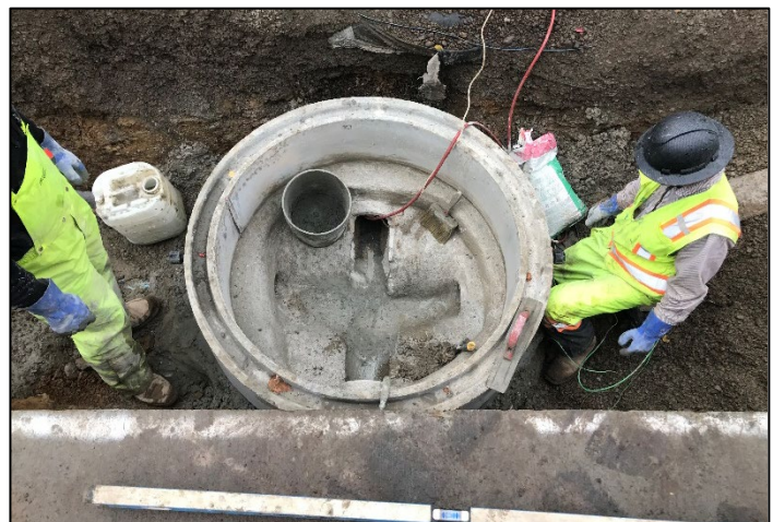
Stormwater manhole installation
