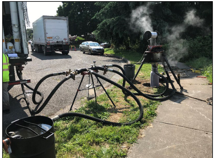
Cured-In-Place-Pipe lining
