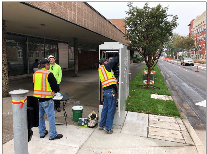
Traffic Signal Controller Installation on 13th Avenue
