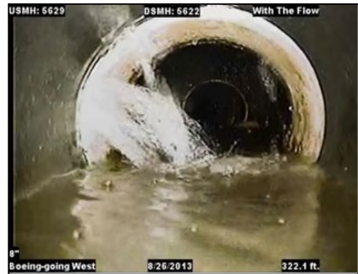
Concrete pipe with excessive groundwater flowing in through open pipe joints.
