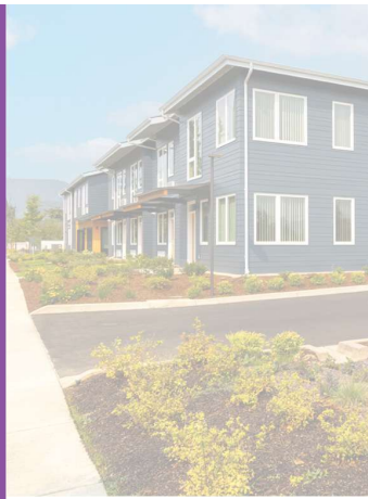
Alma Apartments - construction completed
