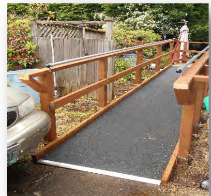
Access ramp, Eugene
