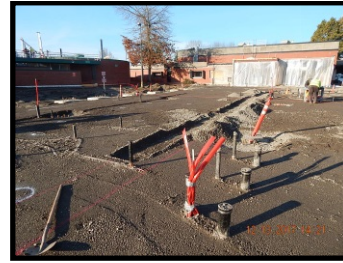
Maintenance Building Expansion
